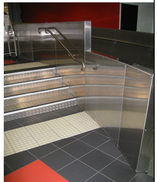
Completed Campbell Street Poly- technic Foyer
