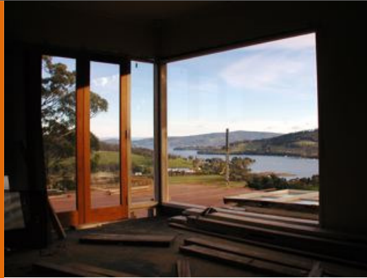
Cygnets house under construction
