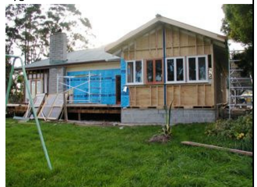
Cygnets house under construction
